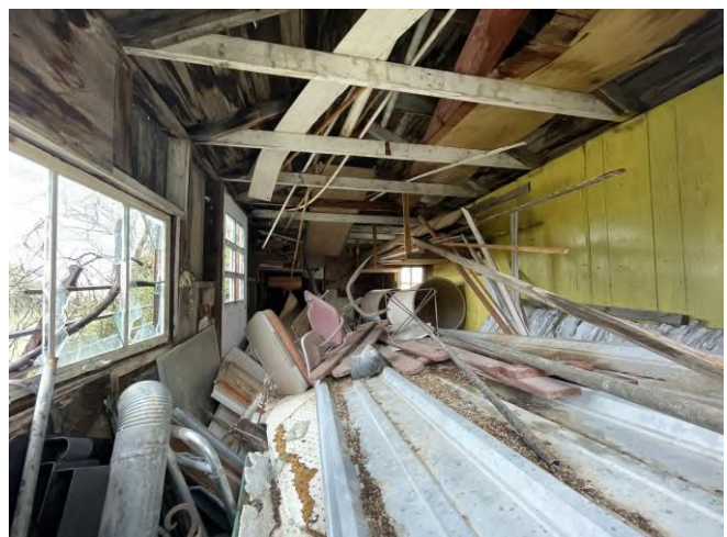
Photo 36: Interior of Building 7.
