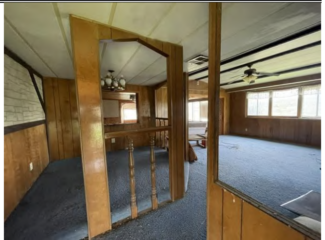
Photo 38: Interior of Building 8.
