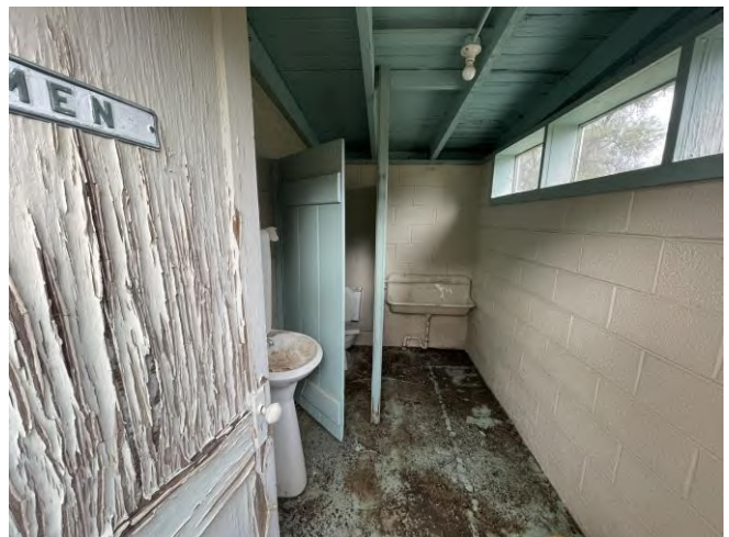
Photo 30: Interior of Building 4.
