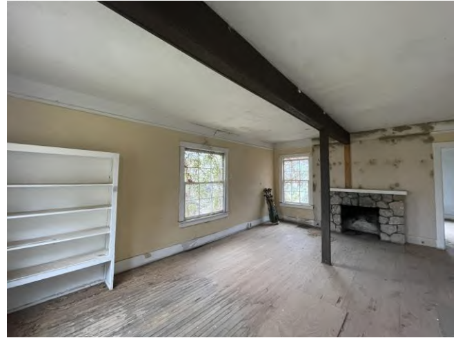
Photo 26: Interior of Building 2.
