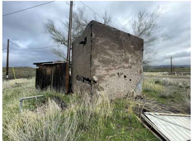
Photo 40: Building 10 – Abandoned well house
