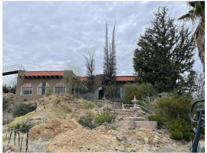
Photo 20: View of Building 1, facing west.
