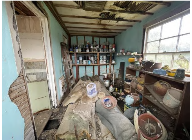
Photo 32: Interior of Building 5.
