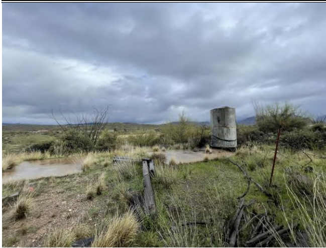
Photo 7: Concrete pad and water storage tank along the southeast Subject Property boundary.
