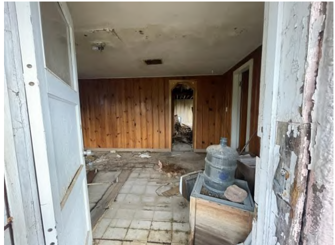
Photo 34: Interior of Building 6.
