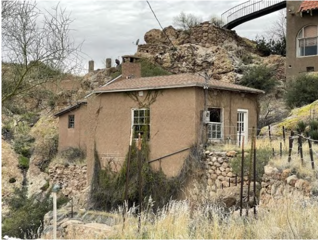
Photo 25: View of Building 2, facing southwest.
