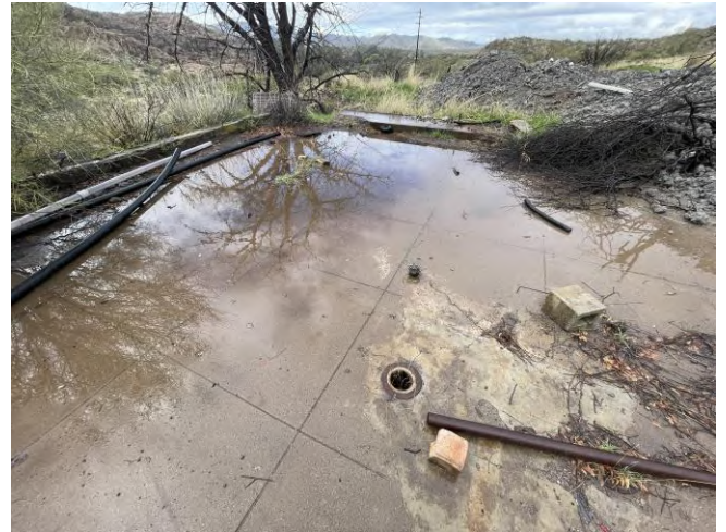
Photo 16: Concrete pad on the west portion of the Subject Property.
