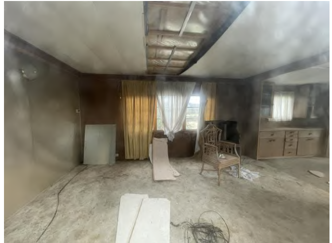
Photo 28: Interior of Building 3.
