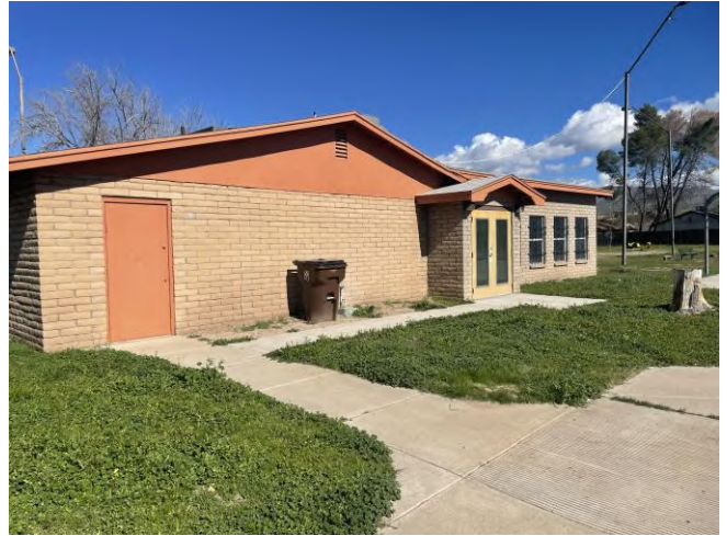
Photo 2: View of the Town Hall building, facing northwest.
