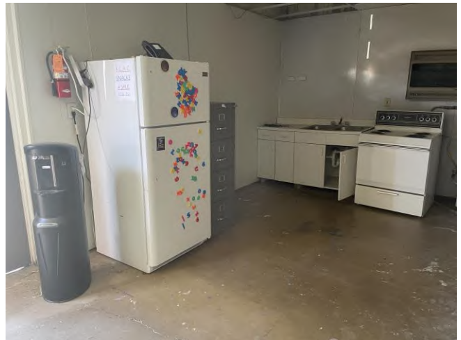
Photo 12: Teen Center kitchen area.
