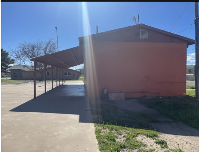
Photo 7: Looking southwest toward the Teen Center building and Town Hall building, beyond.
