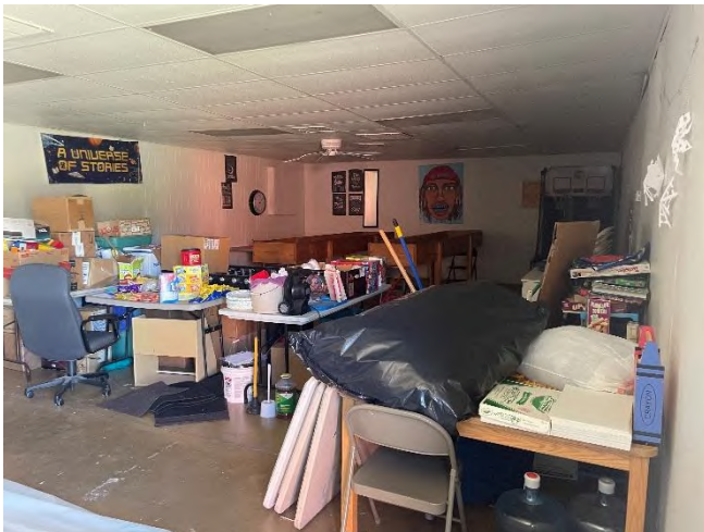
Photo 11: General view inside the Teen Center building.
