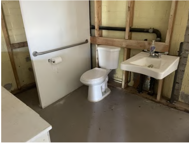
Photo 13: Teen Center restroom area.
