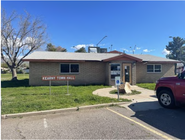
Photo 1: View of the Town Hall building, facing northeast.
