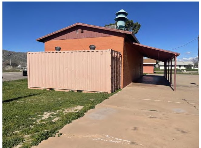
Photo 6: Looking northwest toward the Teen Center.
