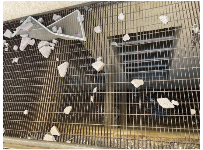
Photo 8: Grate to first floor rear windows.
