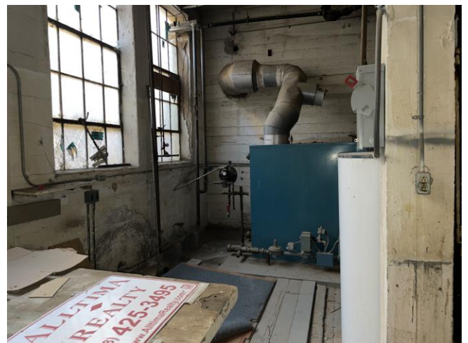
Photo 12: Room J, Boiler room. Floor 1.
