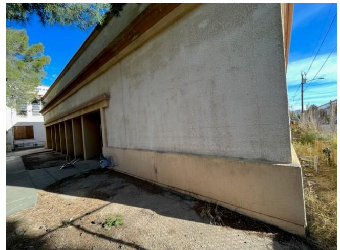
Photo 22: Right face, showing the back of building B.
