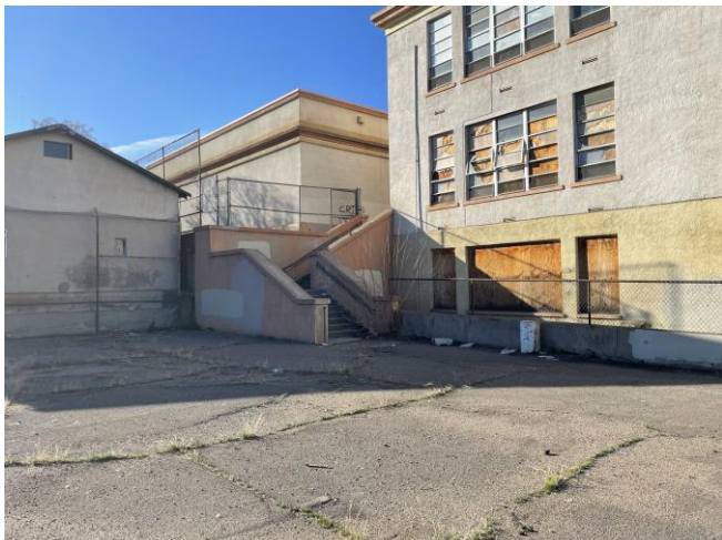
Photo 5: Stairwell on left side leading to the back of school.
