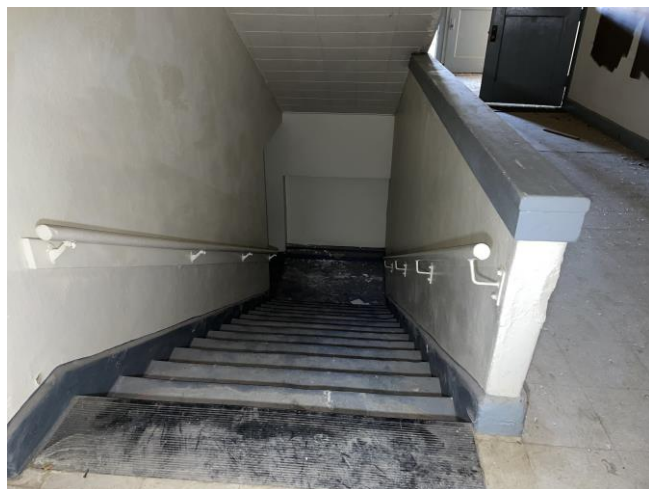
Photo 17: Left side stairwell from floor 1-2.
