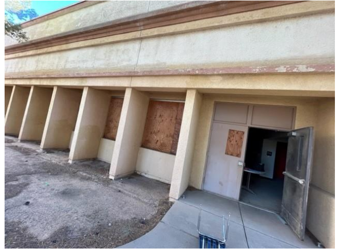
Photo 20: Door used to enter building B, located on the right face of the building.
