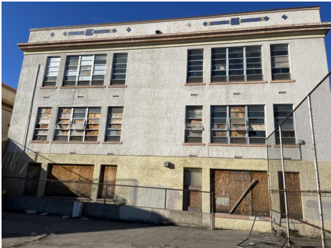
Photo 4: Northeast face of Inspiration school.
