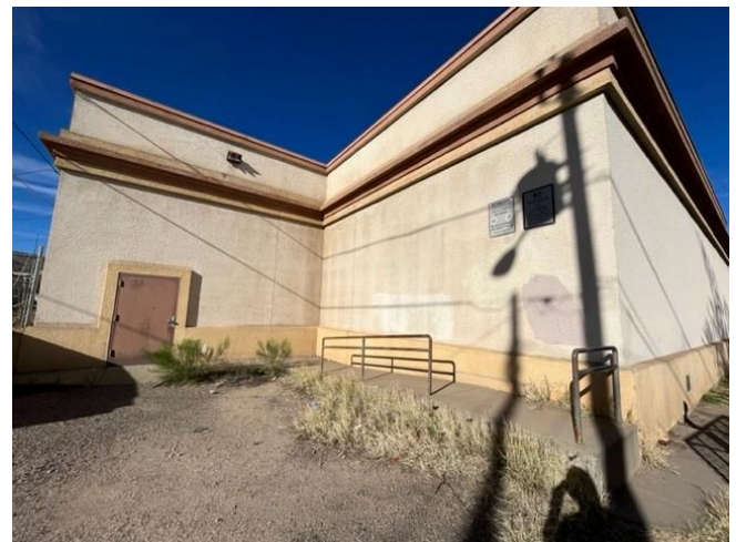
Photo 24: Fuel dispenser near the northwest corner of the Shop building.
