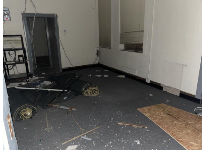
Photo 14: Room Q, Front offices. Floor 1.
