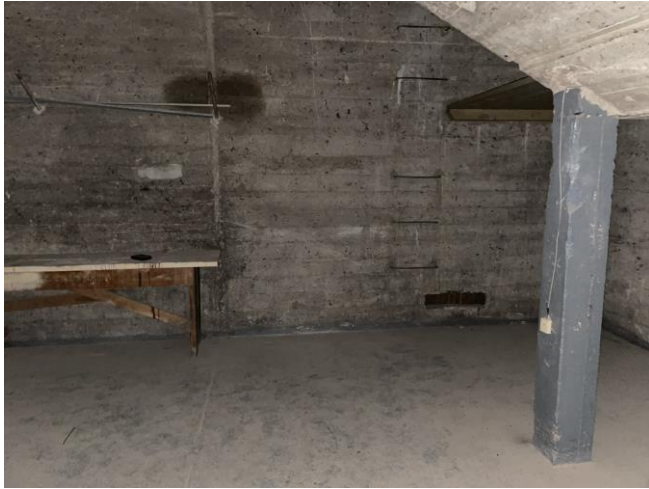
Photo 13: Room K, adjacent to boiler room Floor 1.
